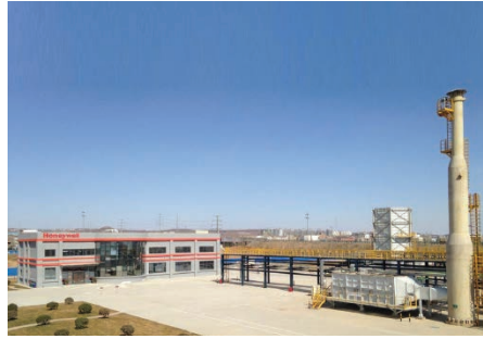
Honeywell UOP Callidus combustion test facility - China
