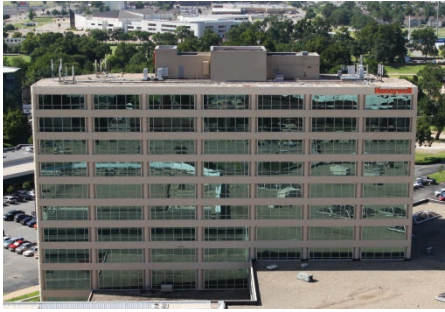
Honeywell UOP Callidus headquarters - Tulsa, Oklahoma. USA
